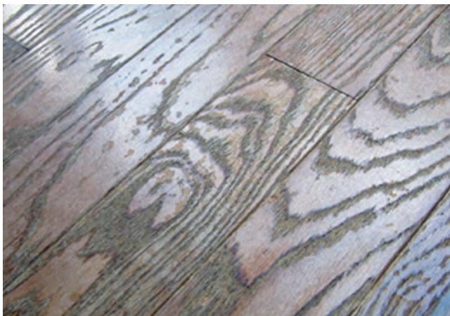
A prefinished timber floor damaged by repeated use of a steam mop cleaner
